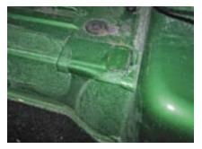
**13.** Clean the mounting surface on the Jeep wheel wells and floor where the bulkhead will be installed. The floor usually has several rough spots where the factory used a seam sealer. We used a 4.5-inch grinder with a wire wheel to knock down the raised areas of the hard seam sealer.
